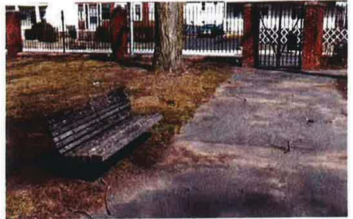
ACCESSIBILITY ISSUES: CRACKS IN PAVEMENT, UNEVEN PAVEMENT
